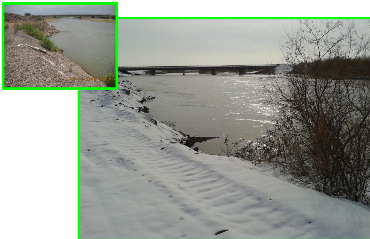
Photo No. 2 : Siltation pond berm Vicinities of Shu River
